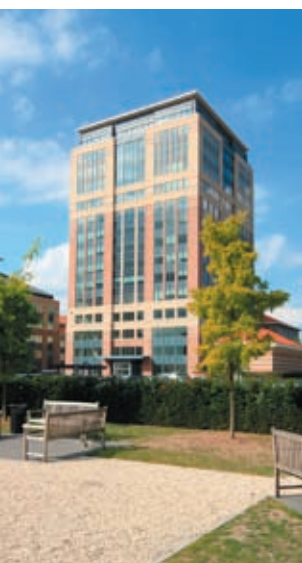
MECHELEN CAMPUS TOWER
