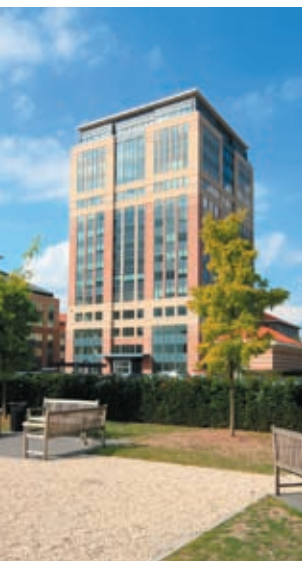
MECHELEN CAMPUS TOWER
